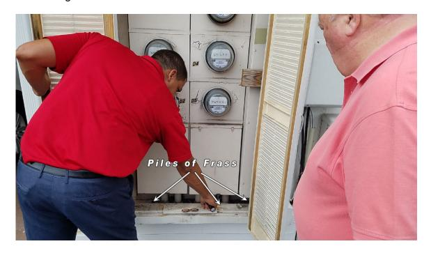
Mike opened up the electrical panel on D Building and pointed out piles and piles of frass, which is evidence of dry wood termites.
