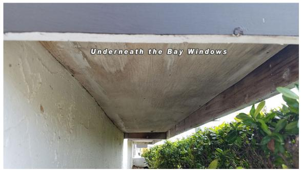
Underneath the first floor bay windows, there is exposed untreated wood.
