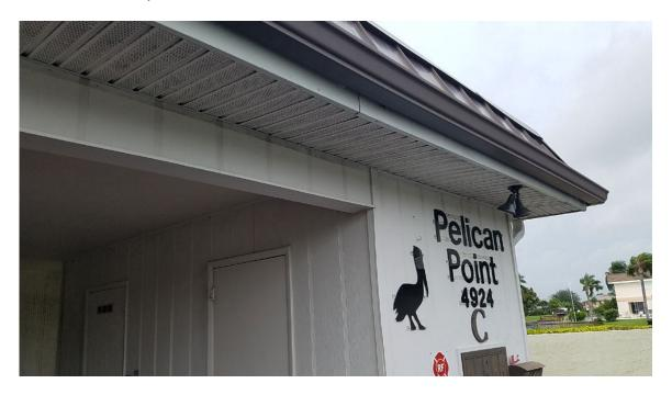
Mike said the soffits are where the majority of the termites are coming in from. Around the building we have these soffits, and behind the soffits, between the floors is wood. Treating the wood between the floors would be a major expense, especially in removing and replacing all the soffits.
