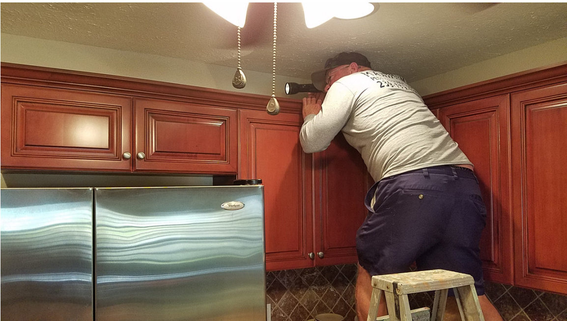
There was FRASS on the tops of the cabinets.
